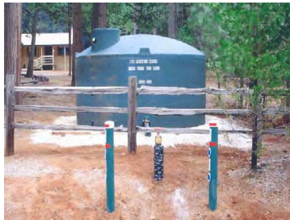
This 5400-gallon tank was installed as a cooperative effort between the fire department and residents. Total cost $3174
