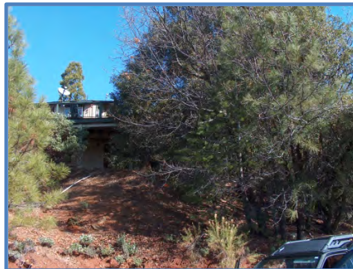
At risk structure
